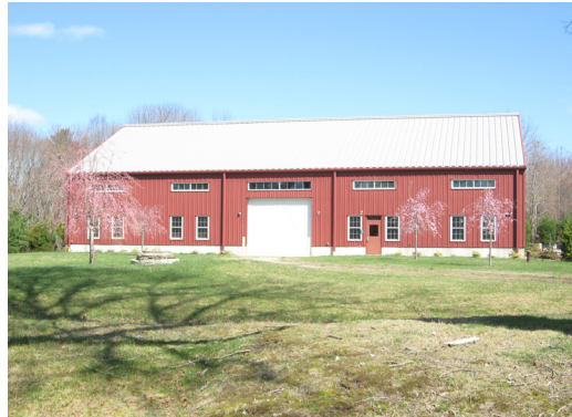
The new Hampton Public Works Garage
